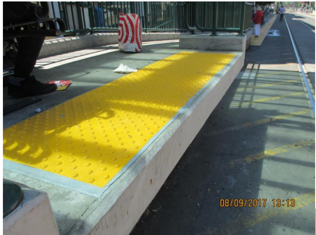
After: Replaced DWT
