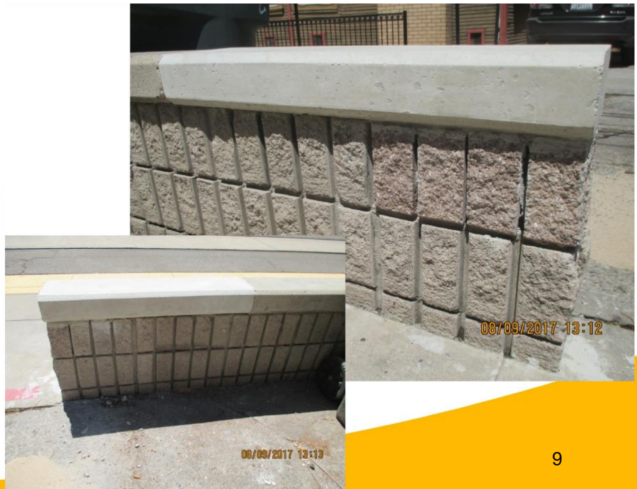
After: Replaced blocks and cap
